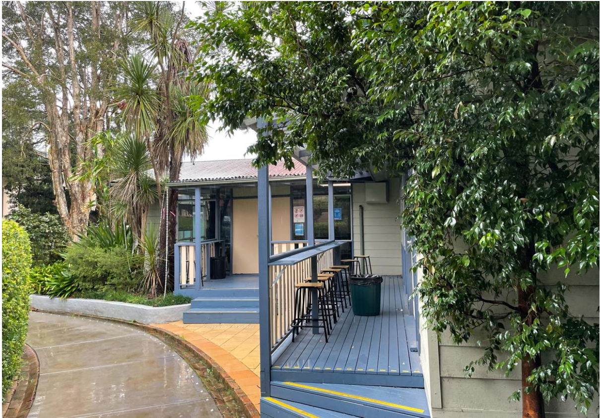
Figure 6: View of eastern extent of existing demountable Salem Building which is to be demolished
