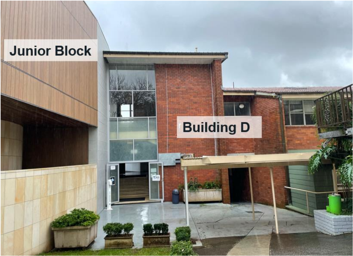
Figure 11: Eastern elevation of the Junior Block which adjoins Building D
