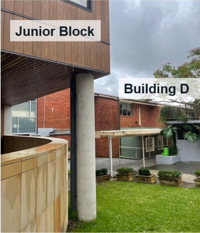
Figure 13: Southern elevation of Building D with the Junior Block in the foreground
