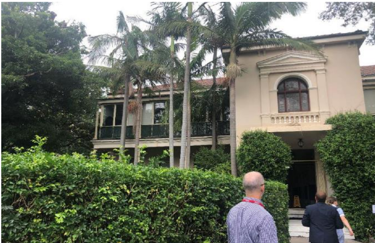
Figure 5: East elevation of Administration Building
