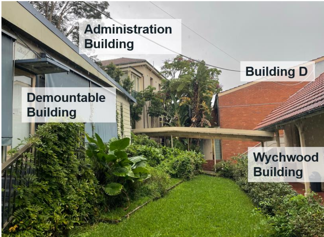
Figure 8: Internal view, noting the demountable building and Building D are proposed for demolition
