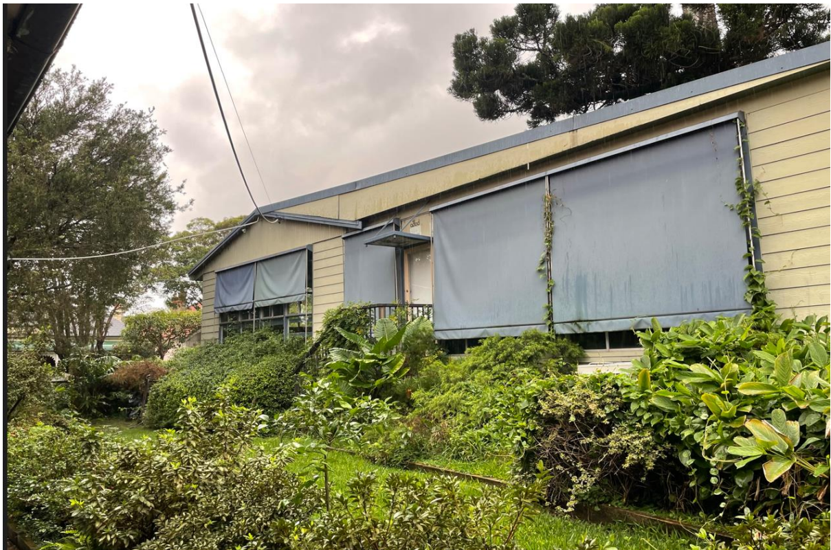
Figure 7: View of western extent of existing demountable Salem Building which is to be demolished
