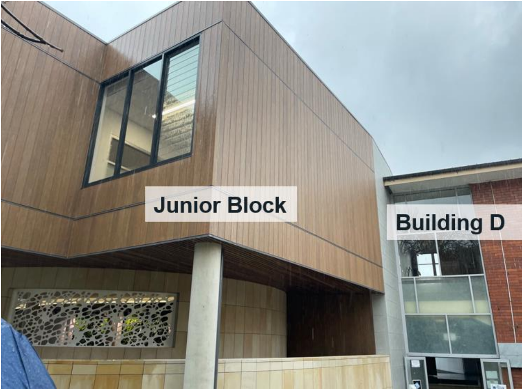
Figure 12: Eastern elevation of the Junior Block which adjoins Building D
